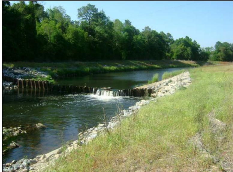
*Figure 2. Wier on the Montlimar Canal. Note rocks to repair bank erosion*
